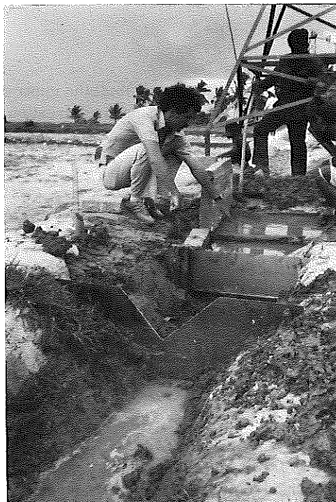
Fig. 4 V-notch flow measuring system
