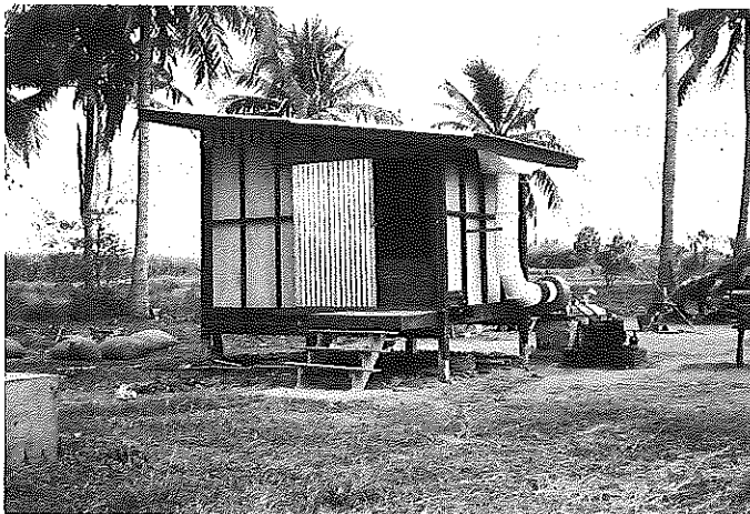
Fig. 5 Photograph showing another view of the solar hut.
