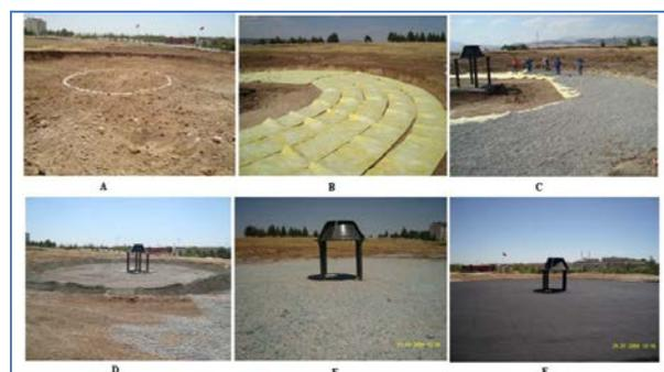
Fig. 6. Pictures showing the construction steps of ground of the Abdulceli prototype (A ground floor, B Aluminum folio with glass wool, C Gravel laying, D Sand, E Glass laying, F Asphalt paved) [11].
