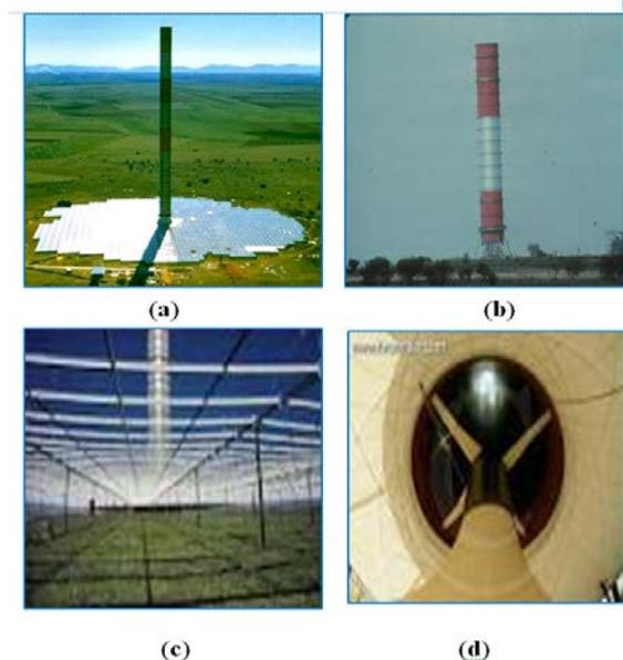
Fig. 2. (a) Solar chimney power plant in Manzanares, Spain; (b) chimney tower; (c) collector; (d) wind turbine; [6].
